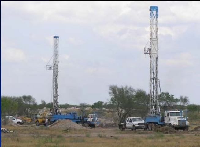
Wellfield Development drilling activities. (above)
