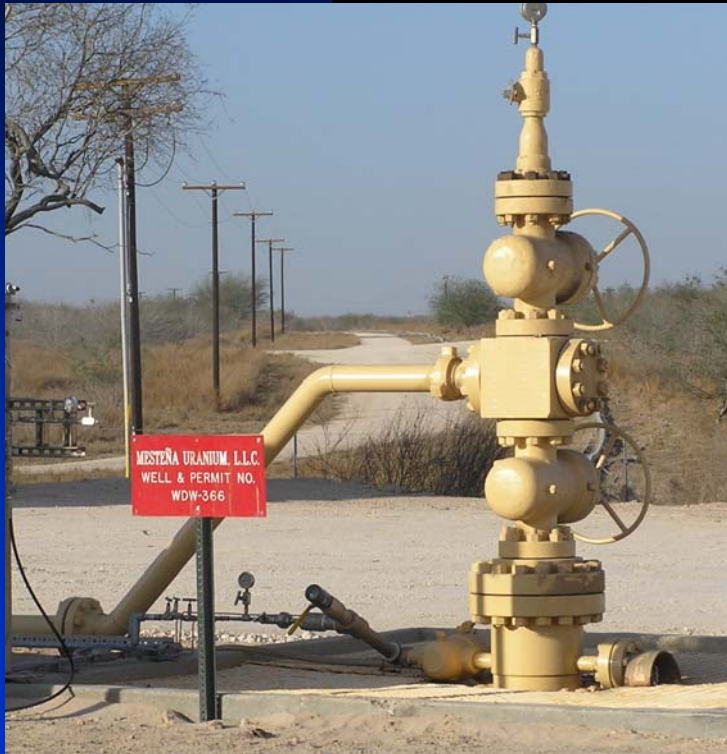
A permitted Class I disposal well for process effluents
