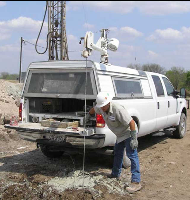
Open hole logging of a drill hole. (above)
